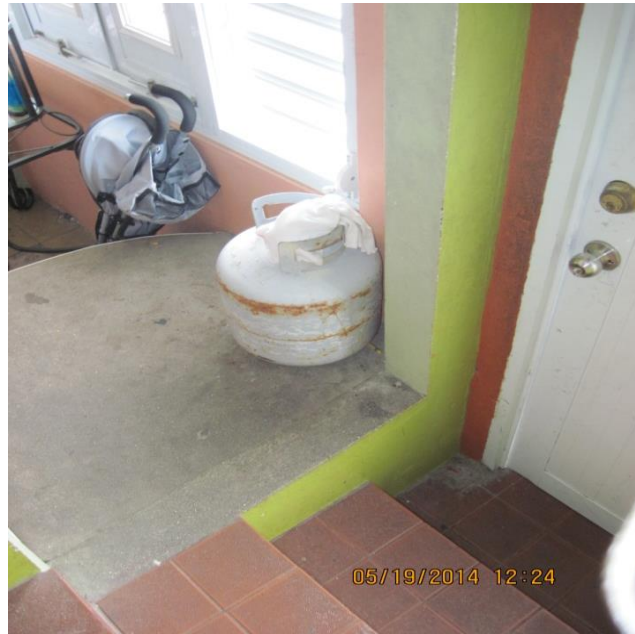
Photograph 9: A rusted propane gas tank inside the entrance to the provider's home. The tank could leak or be turned on and cause a catastrophic explosion.
