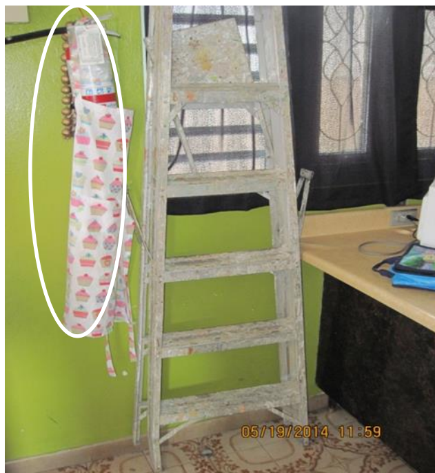
Photograph 8: A fire extinguisher covered by an apron, and an unsecured tall metal ladder leaning on a wall of the children’s play area.
