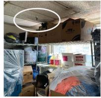
Photograph 5 (left): Kitchen fire suppression system did not have monthly inspections. Photograph 6 (center): Fire extinguisher did not have monthly inspections. Photograph 7 (right): Sprinkler head obstructed by storage boxes.
