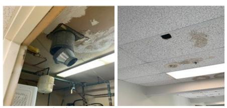
Photograph 3 (left): Metal duct dangling from ceiling. Photograph 4 (right): Damaged ceiling tile.
