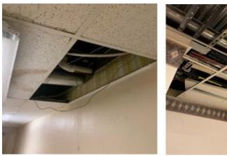
Photograph 1 (left): Missing ceiling tiles. Photograph 2 (right): Missing ceiling tiles.
