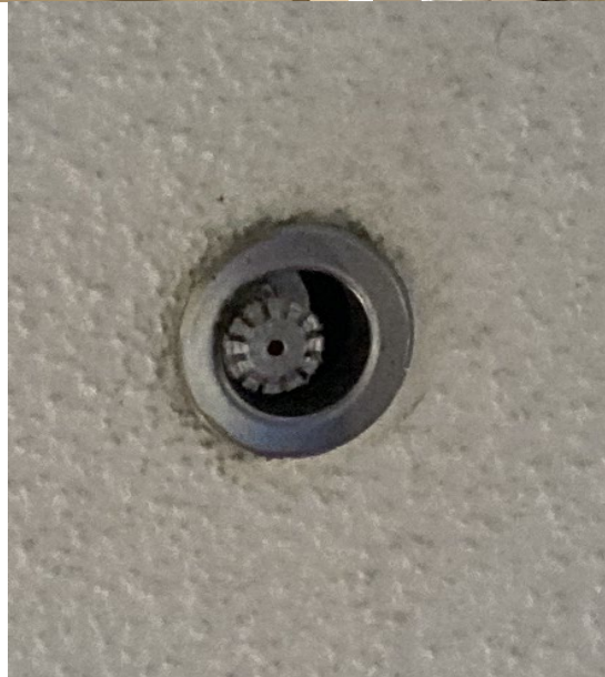
Photograph 4 (upper left): Boxes are too high and obstruct sprinkler.
