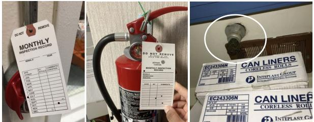
Photograph 5 (left): Kitchen fire suppression system did not have monthly inspections. Photograph 6 (center): Fire extinguisher did not have monthly inspections. Photograph 7 (right): Sprinkler head obstructed by boxes.
