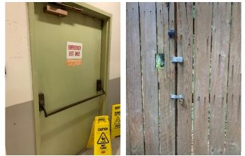
Photograph 1 (left): Door marked as emergency exit led to patio with locked gate. Photograph 2 (right): Locked gate in patio with no exit path.
