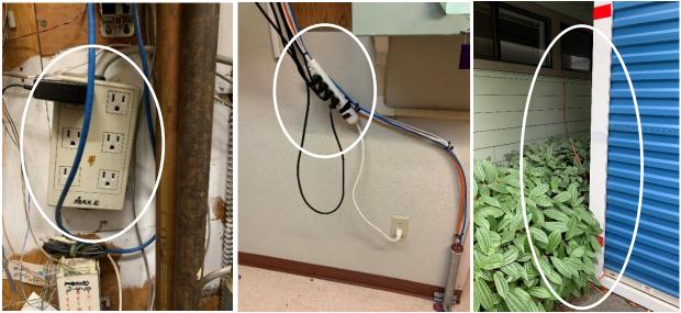
Photograph 10 (left): Power strip mounted to a wall. Photograph 11 (center): Power strip mounted to voice and data cables. Photograph 12 (right): Unallowable use of extension cord connected to item in locked storage container (nursing home management did not have access to storage container).
