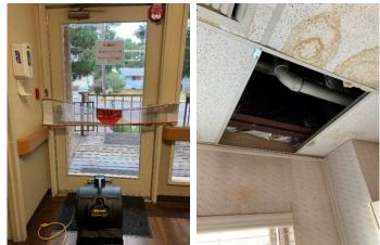
Photograph 3 (left): Pathway to exit blocked by fan. Photograph 4 (right): Hole in smoke partition from missing ceiling tile.
