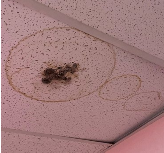
Photograph 1: Water Damage
