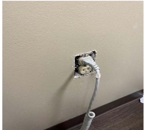
Photograph 2: Exposed Electrical Outlet
