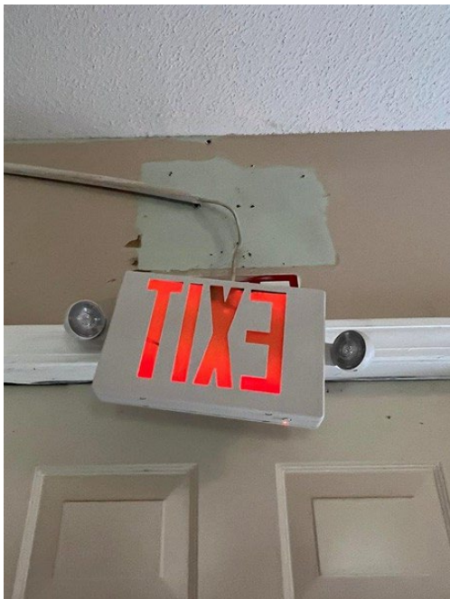
Photograph 13: Exit Sign Hanging From Loose Electrical Wiring
