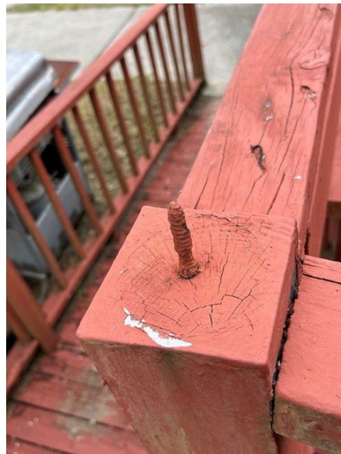
Photograph 14: Screw Protruding From Handrail
