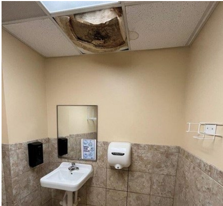
Photograph 5: Water Damage
