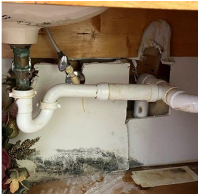
Photograph 8: Water Damage and Mold
