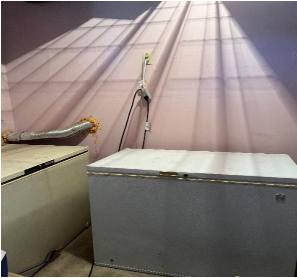
Photograph 11: Two deep freezers plugged into the same garage outlet creating fire hazard
