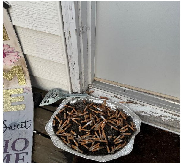
Photograph 14: Smoldering cigarettes in disposable pan, kept on wooden deck, some noted to have missed the pan and scattered along wooden door frame and deck creating a fire hazard
