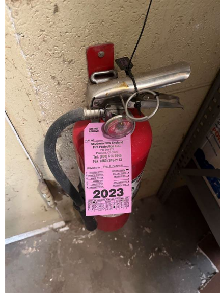
Photograph 6 (left): Wasp nest obstructing sprinkler head. Photograph 7 (right): Fire extinguisher last inspected in 2023, instead of monthly as required.
