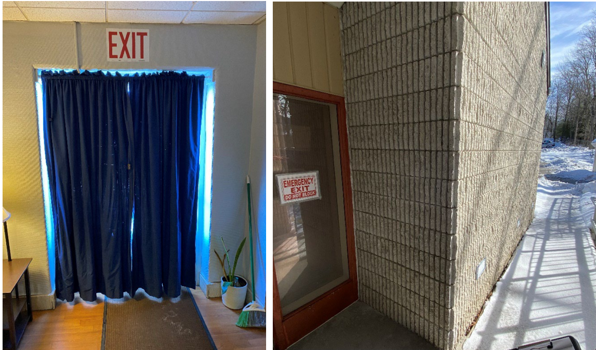
Photograph 4 (left): Pathway to exit blocked by curtain and nonilluminated exit sign. Photograph 5 (right): Emergency exit and egress path covered by ice and snow. Snow piled at bottom of path.
