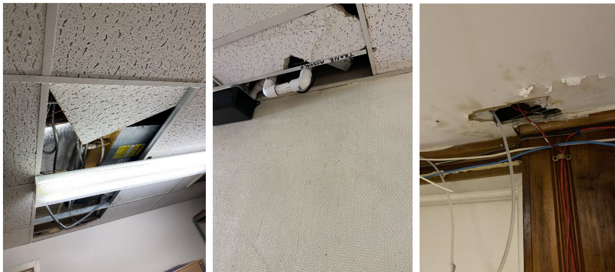
Photograph 1 (left): Misplaced ceiling tile. Photograph 2 (middle): Broken ceiling tile. Photograph 3 (right): Hole in the ceiling.
