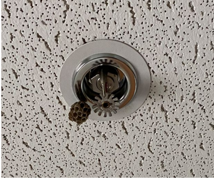
Photograph 6 (left): Wasp nest obstructing sprinkler head. Photograph 7 (right): Fire extinguisher last inspected in 2023, instead of monthly as required.
