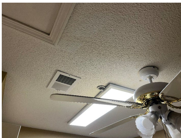
Photograph 9: Partially obstructed sprinkler head.
