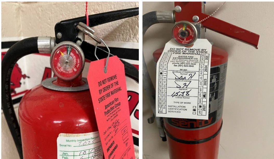
Photograph 7 (left): Fire extinguisher not properly charged.
