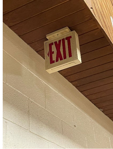
Photographs 3 and 4: Non-illuminated emergency lighting.
