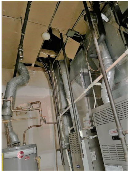
Photograph 5: Hole in ceiling in mechanical closet.
