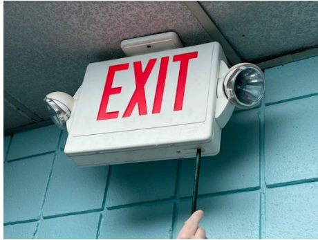
Photographs 3 and 4: Non-illuminated emergency lighting.
